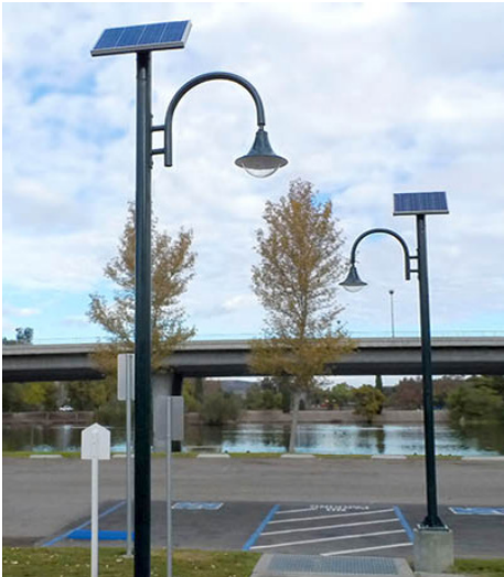
Solar powered pedestrian lights
