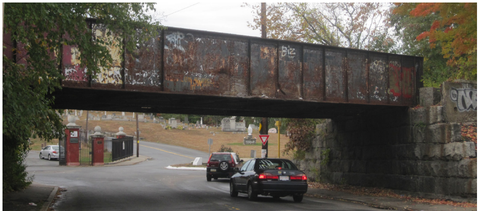
Existing Manchester Street Bridge exterior condition
