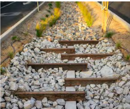
Rail stormwater runoff attenuators
