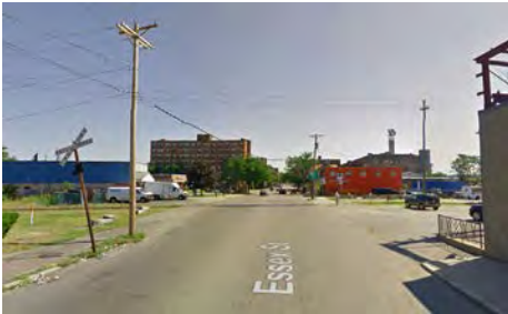
View of at-grade crossing at Essex Street
