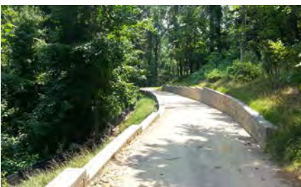
Accessible ramp along slope
