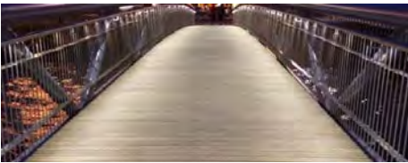
Pedestrian bridge handrail lighting
