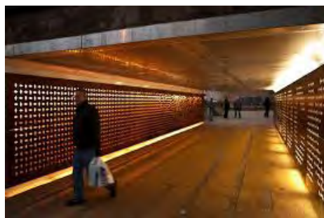
Bikcycle/pedestrian underpass lighting
