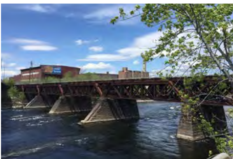
Merrimack River Bridge
