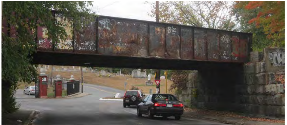
Existing Manchester Street Bridge exterior condition
