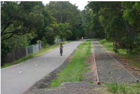
Existing Tracks Parallel to New Trail
