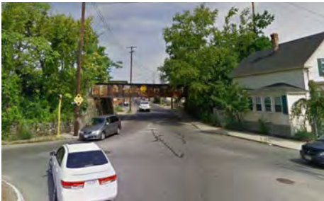
View of elevated Manchester Street Bridge
