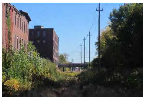
Existing Lowell Street Bridge
