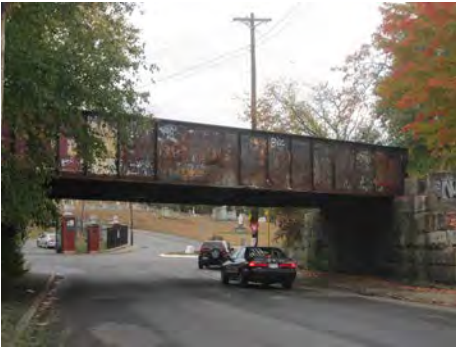
Manchester Street Bridge
