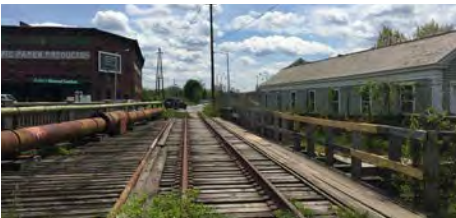
B&M Railroad Bridge over the North Canal
