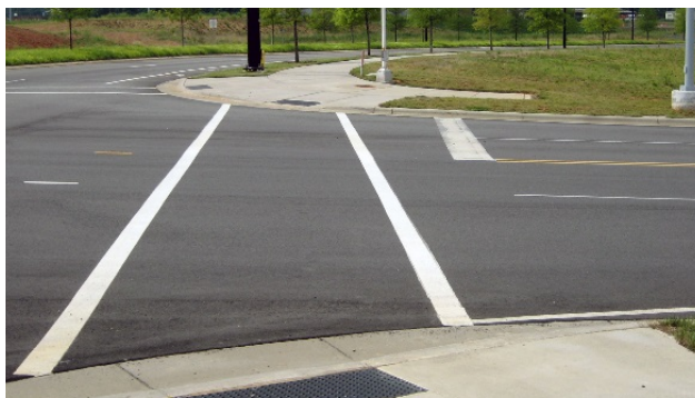
Figure III.19. Parallel Line (or Traverse Line) Crosswalk is less visible to drivers, particularly at night.
