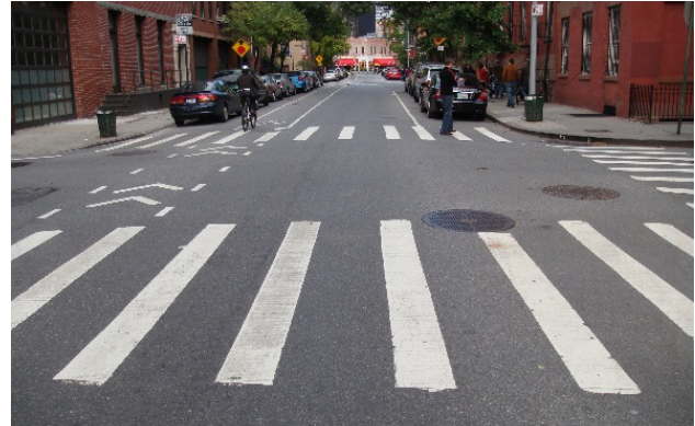
Figure III.20. Bar or Zebra Crosswalks improve pedestrian safety and are more visible to drivers.
