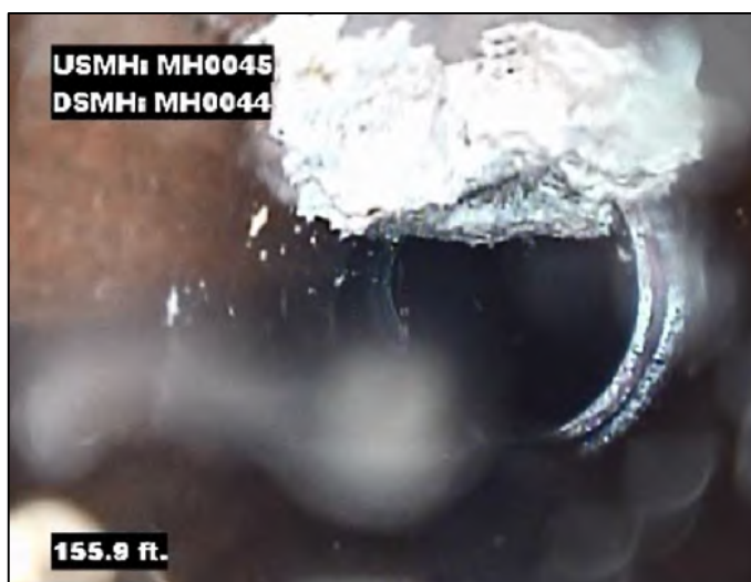
Figure 1-1: FOG Buildup in a Lawrence Sewer Pipe
