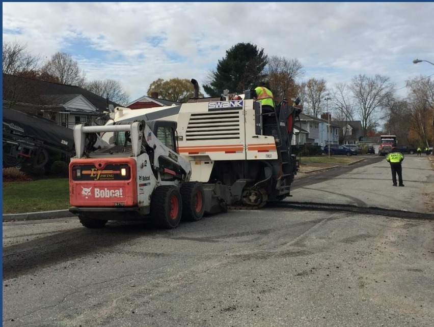
Columbia Gas crews mill trenches in Lawrence.
